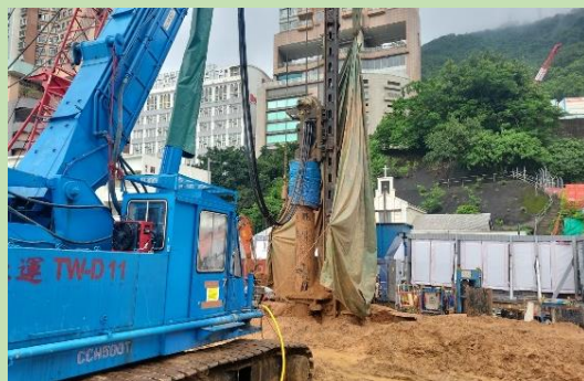
升降機塔打樁工程 Pilling Works for Lift Tower Construction
