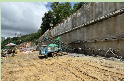
擋土牆打樁工程 Pilling Works for Retaining Wall
