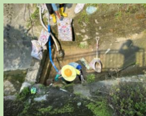
清理排水設施 Clearing the Existing Drainage Facilities
